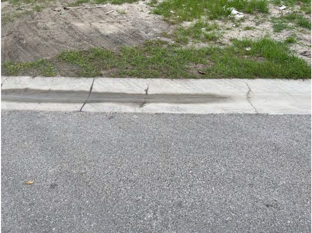
Multiple gutter cracks next to 13447 Seabridge
