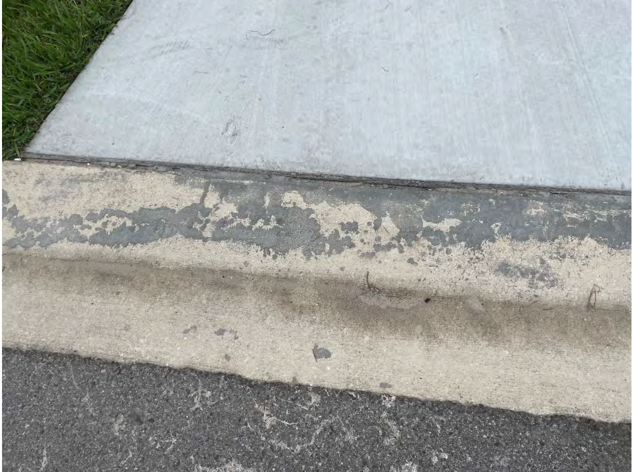
Excess concrete 13826 Moosehead driveway
