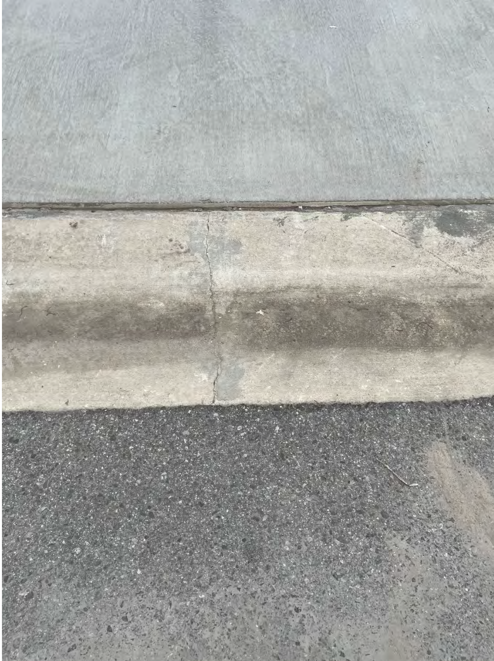
Gutter crack driveway at 13850 Moosehead
