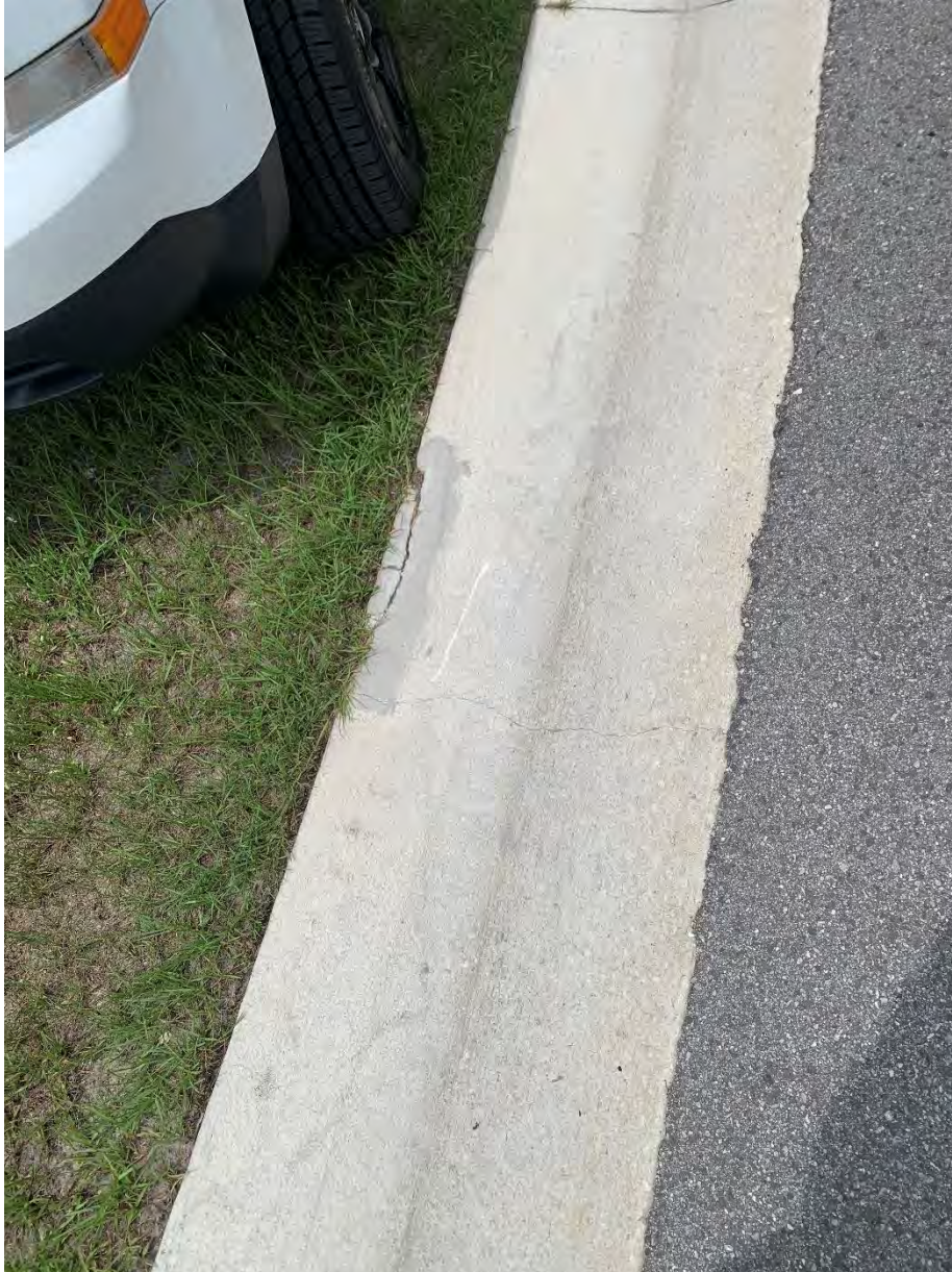
11 – Gutter damage on Sea Bridge
