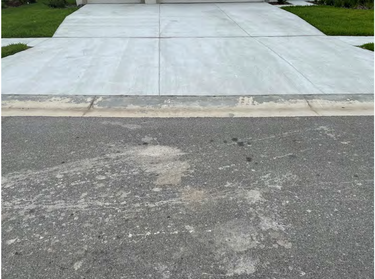
Excess concrete 13826 Moosehead driveway
