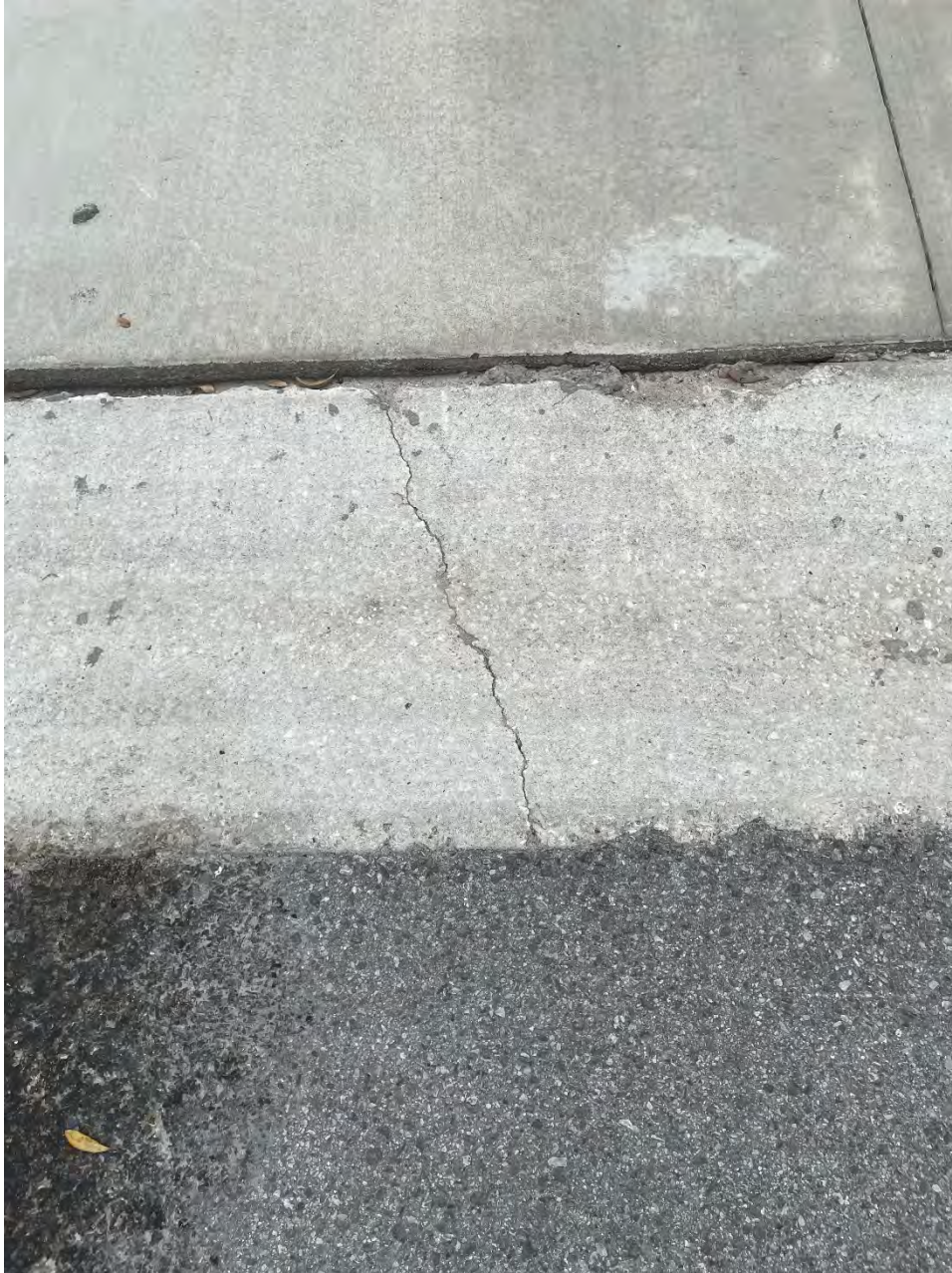
Gutter crack at driveway 13447 Seabridge
